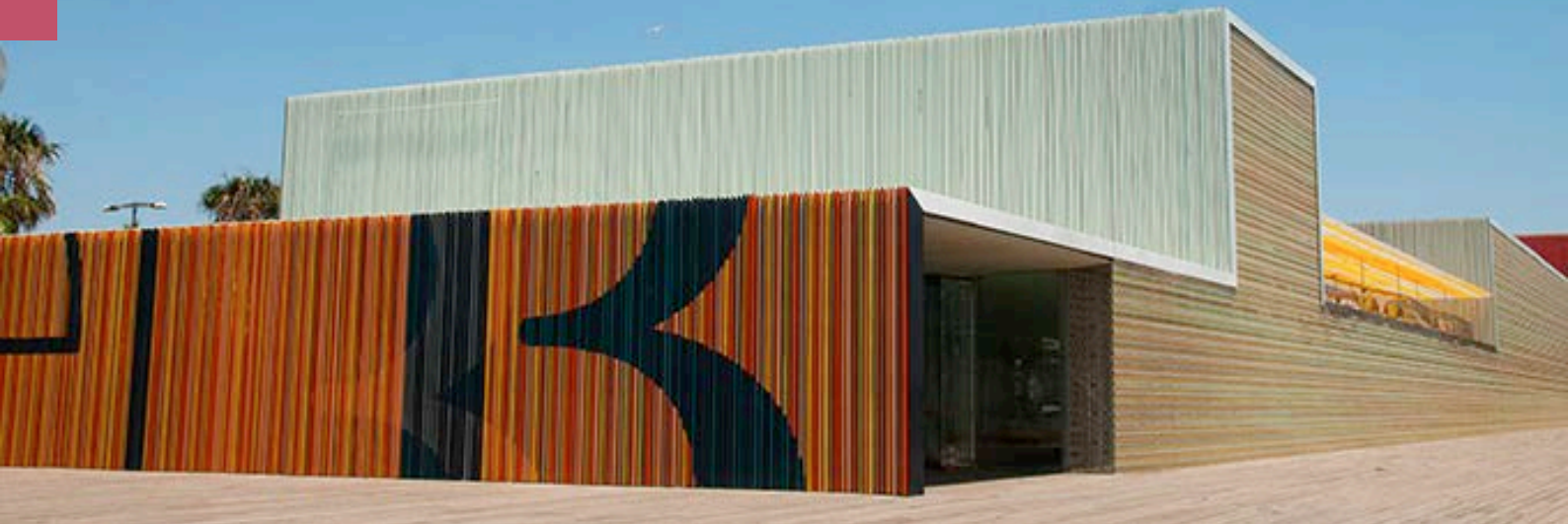
Cartagena's Auditorium and Convention Hall. Its location near the harbour and the sea inspired its design.
